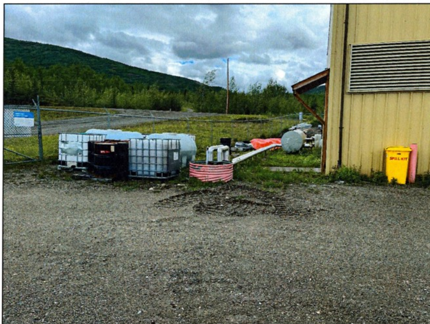
Figure 2: Glycol coolant stored uncovered and unsecured.
