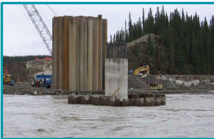
3.9-01 Cofferdams used in construction of bridge piers.
