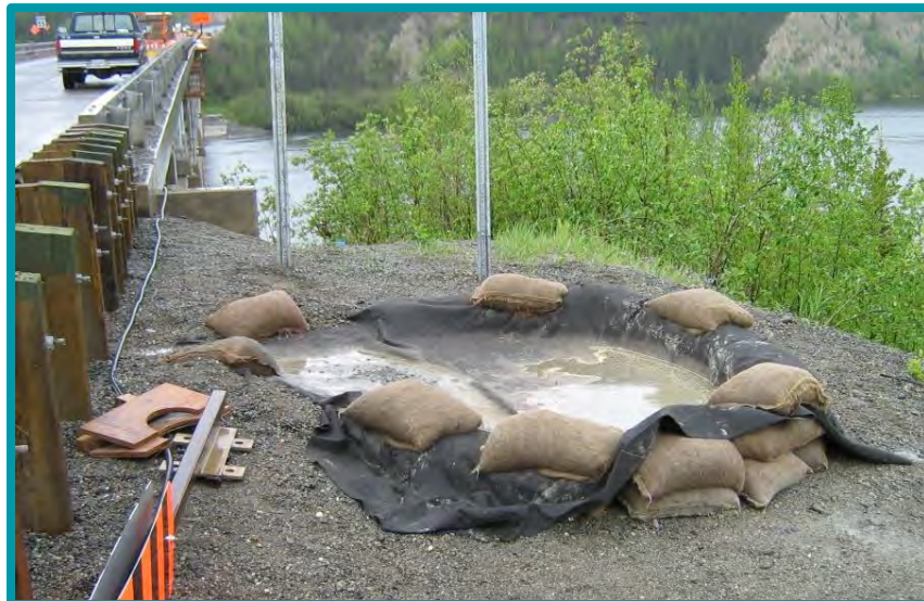
2.1.8-03 The size of a sediment trap depends on the volume of water that will be generated and sediment settling rate. This trap, while small, was built to contain a small volume of concrete cooling water, and was completely adequate for the job.
