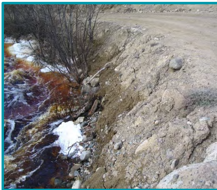
2.1.1-01 An unprotected stream bank that is being eroded by high water.
