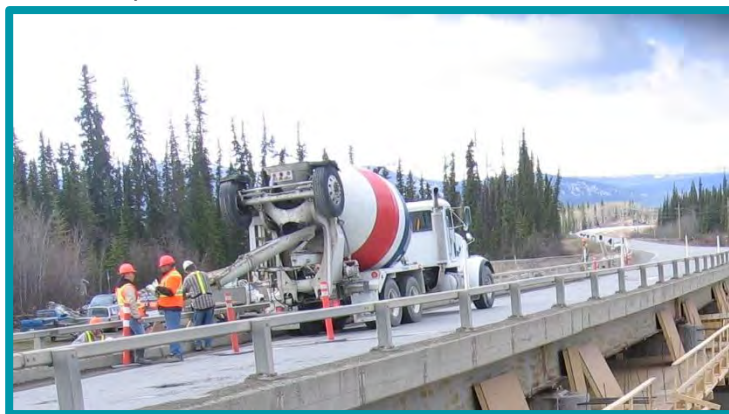
2.2.2-01 A sturdy work platform constructed below this bridge allowed easy access to the superstructure, but it also helped catch debris and keep uncured concrete from falling in the water.
