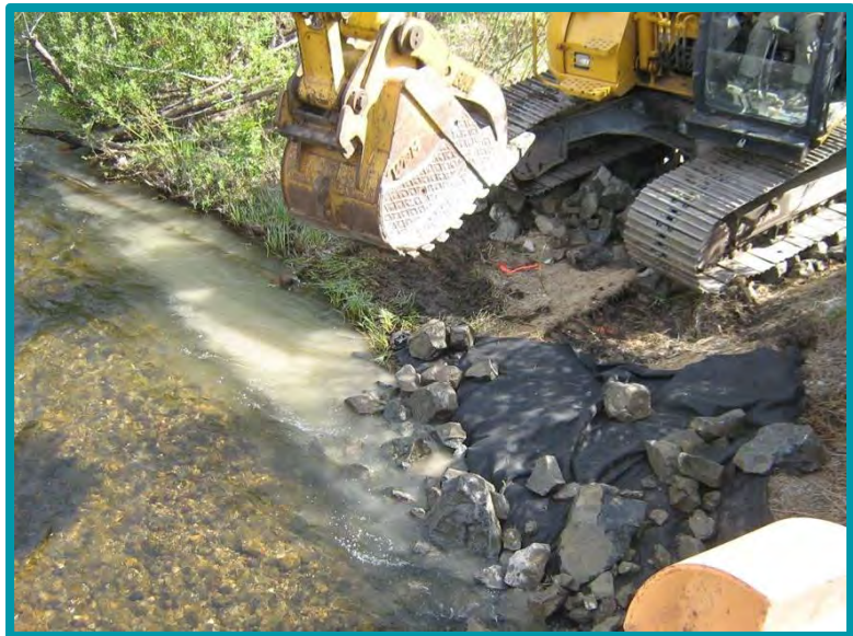
3.1-01 The rock being placed in this stream is covered with sediment and is depositing silt in the stream. It should have been washed prior to careful placement in the stream.
