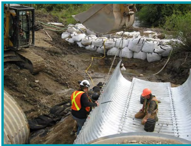
3.8-08 Same site - the work area is dry and the culverts extensions are being attached.
