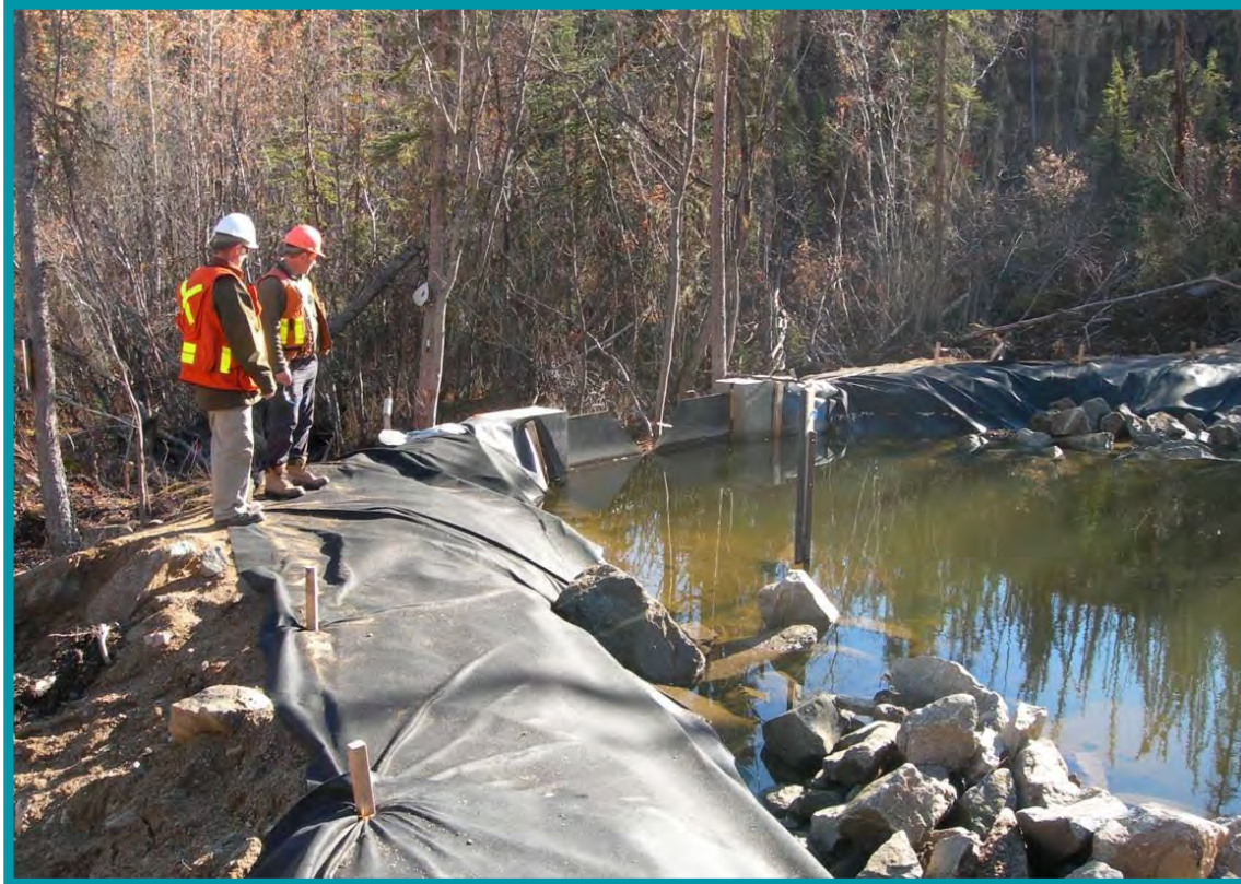
2.1.8-05 This is a well-constructed and designed sediment trap with a passive overflow.
