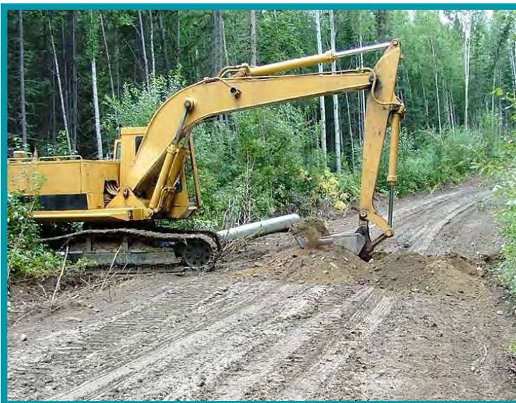
3.3-02 Installation of a culvert to provide cross drainage.
