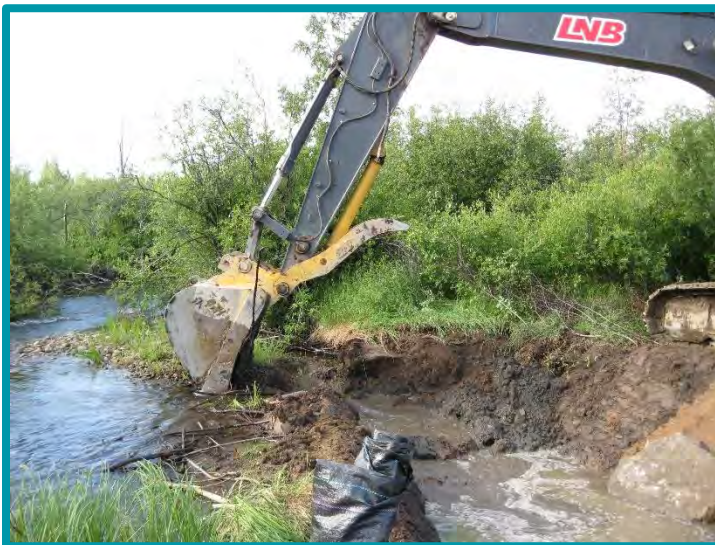
3.8-04 Same site - the downstream earth plug is being removed.
