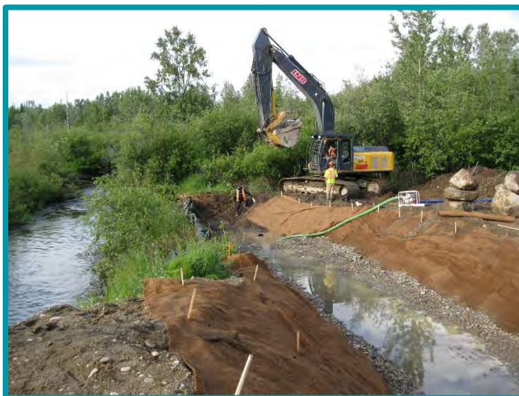
3.8-03 The project in the following six photos involved lengthening two existing culverts at Watson Creek. To complete the work, the creek had to be diverted so the culvert extensions could be completed in the dry. This photograph shows the diversion channel on the right and Watson Creek on the left. The banks are lined with jute fabric to protect them from erosion. The new channel is being washed and the sediment-loaded water is being pumped out into the vegetation.
