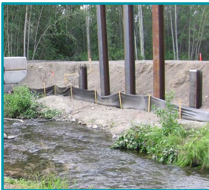
2.1.7-03 This silt fence was installed along a creek as a perimeter fence to keep loose material from rolling into the water.
