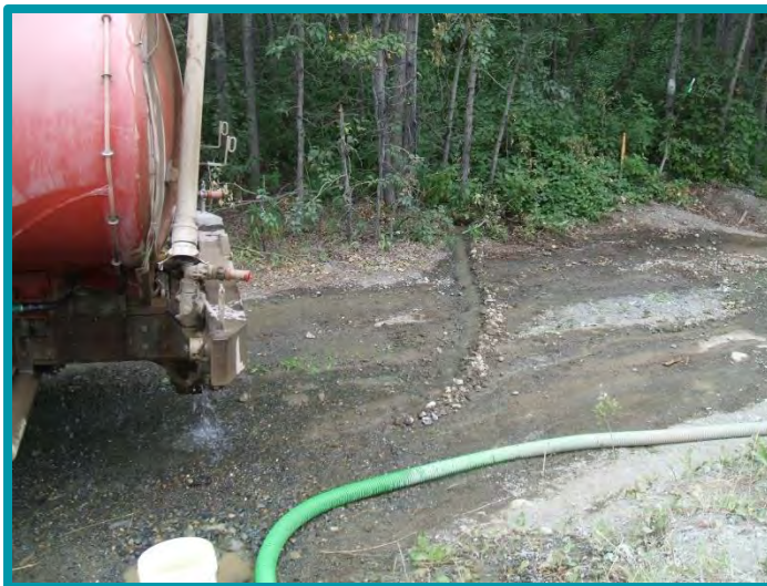
3.1-02 A simple diversion was created to guide runoff into the vegetation, rather than the stream. Sometimes it's the little things that make a big difference.
