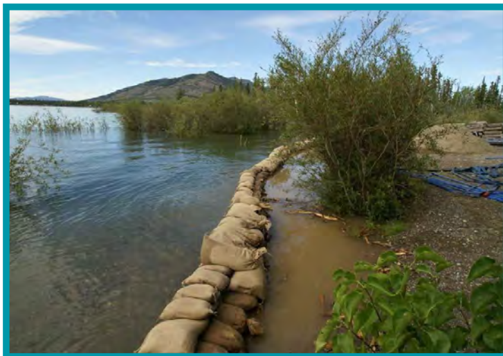
3.9-02 Sand bags being used to protect an eroding lake shore. Note clear water in the lake and the turbid water along the shore.
