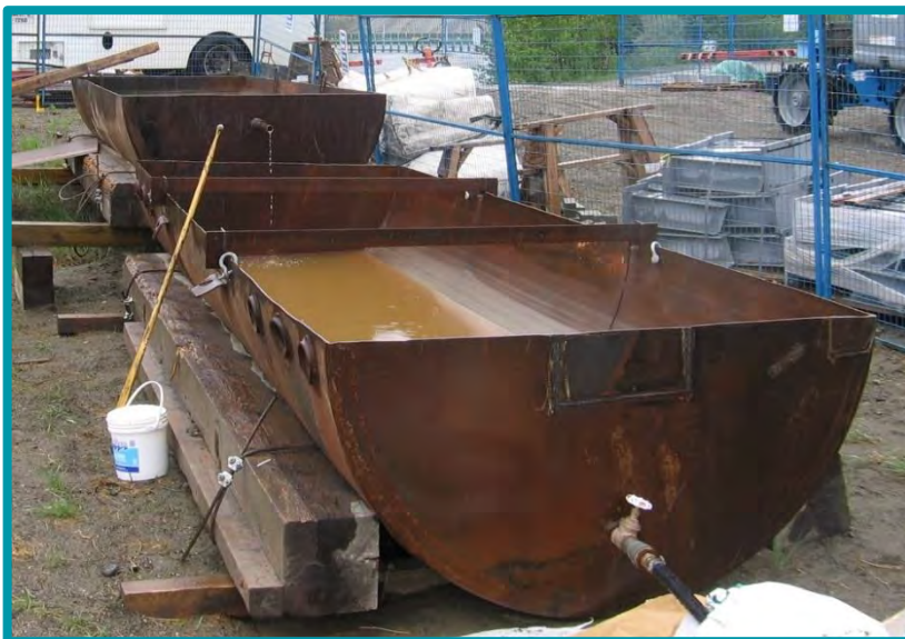
2.1.8-02 Creative use of an old fuel tank as a sediment settling system. The upper container receives the sediment-laden water and has a passive overflow to the lower container, which has an outlet controlled by a valve.
