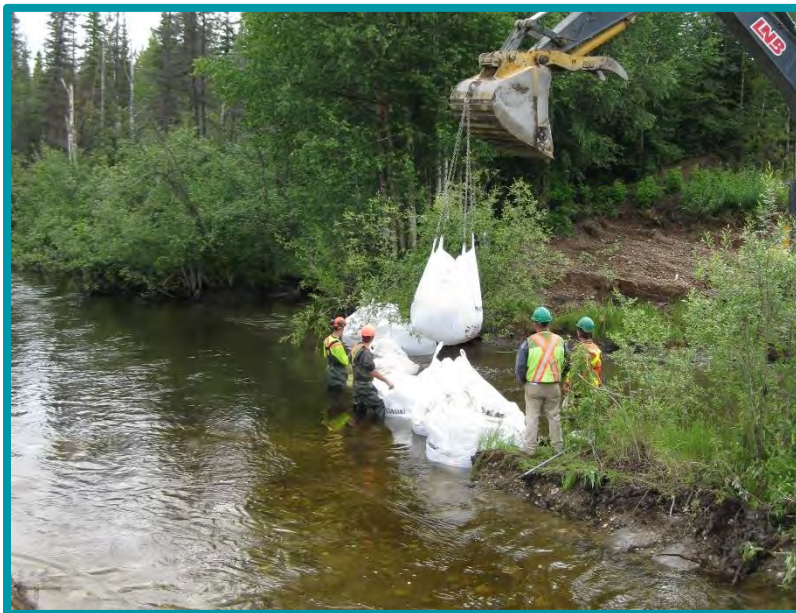
3.8-06 Same site – Watson Creek is being blocked off with large sand bags and the flow is captured by the diversion channel (foreground).
