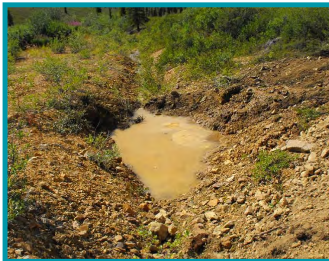
2.1.8-04 A small excavated sump built to collect runoff from an exploration trench. Simple, but effective.
