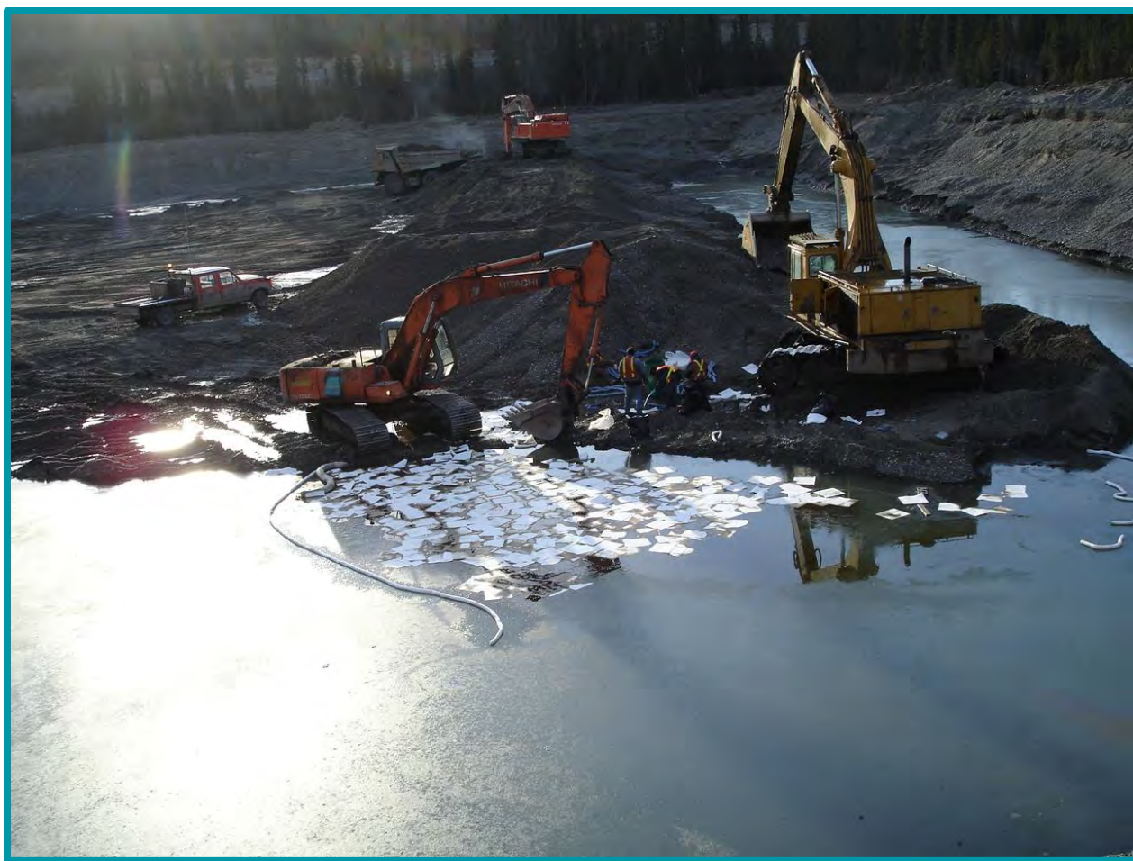
2.2.1-03 Emergency response. An oil spill occurred on this small lake during gravel extraction activities when a crack developed in the oil reservoir of an excavator. Booms are being deployed to contain the spill, and oil on the surface is skimmed off using absorbent pads. Ice on the lake helped contain the spill.
