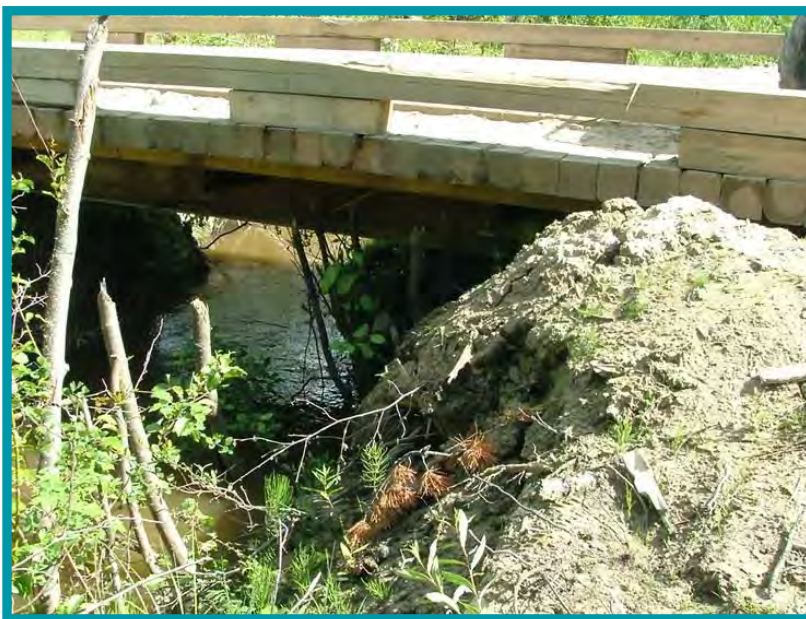
3.5-03 The abutment of this clear-span bridge should have been protected with riprap. Embankment collapse and sediment release are imminent.
