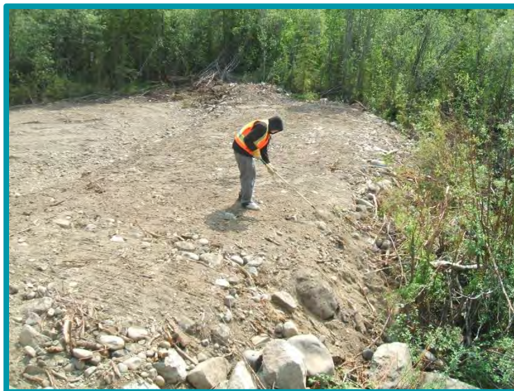
2.1.2-06 A small area next to a creek is being raked in preparation of seed application.
