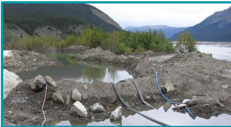
2.1.8-01 This sediment trap contains water pumped from isolated in-stream work areas created to construct a new bridge pier. This sediment trap has a passive overflow near the top of the picture. Clear water exits the overflow and passes through vegetation before re-entering the stream.
