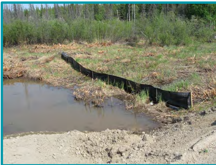
2.1.7-02 This silt fence should have been installed at the bottom of the disturbed slope rather than in the undisturbed vegetation. Currently it is non-functional.
