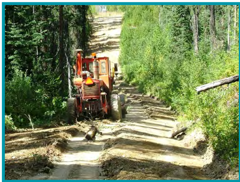
3.3-03 Proper sloping, crowning, and ditch placement on this road is creating good drainage and a stable roadbed.
