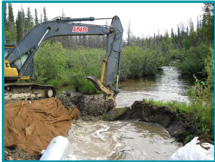
3.8-05 Same site - the upstream earth plug is being removed.
