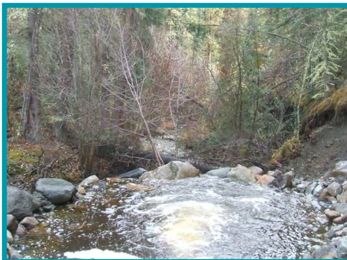
3.8-02 Same site as above - the pumped water was released downstream of the work site in an excavated depression that was lined with rock to slow the flow velocity and trap sediment. This picture shows the pumped water bubbling up and overflowing the rock lined area. The actual creek is in the background.
