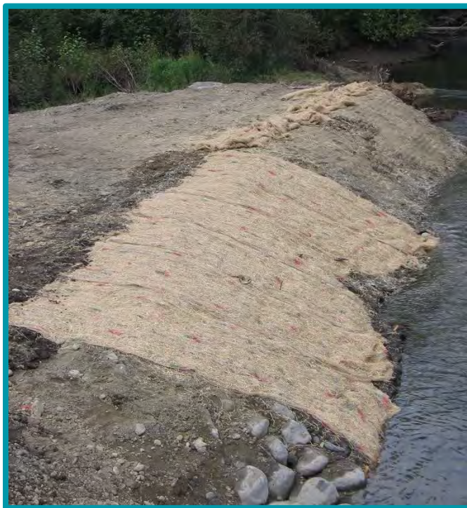
2.1.4-01 A manufactured erosion control product composed of straw and jute mats being installed along a creek. The surface was seeded before the matting was unrolled, and later on willow cuttings were planted at the water's edge.
