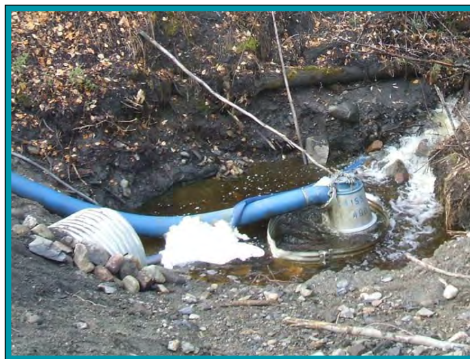
3.8-01 A pumped diversion showing the water intake. Even for this small stream, pumping its entire flow across the work site required large volume pumps.
