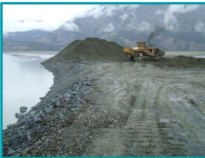
3.1-03 This stockpile of loose material should have been covered with plastic or geotextiles to avoid sediment runoff into the river. Depending on how and when the material was to be used, it also should have been stockpiled away from the river.
