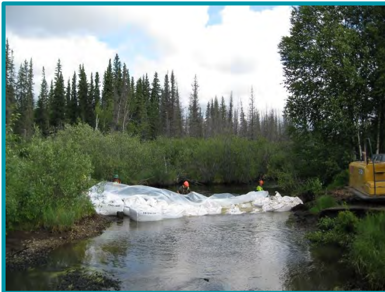
3.8-07 Same site - the sand bags are covered with plastic on the upstream side of the diversion. The plastic is anchored on the bottom with rocks to hold it in place and to seal the stream blockage.
