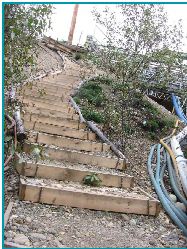
2.1.1-04 These steps were created for easy access from a steep bank down to the river. They also avoid unnecessary erosion of the bank. Smart planning can avoid problems down the line.
