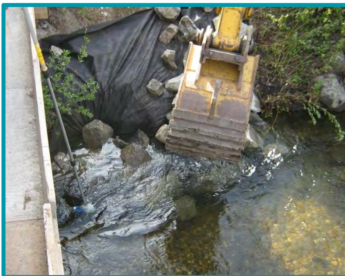
3.10-01 Careful placement of clean rock along a stream bank. A water sample is being collected to measure the turbidity caused by sediment release.
