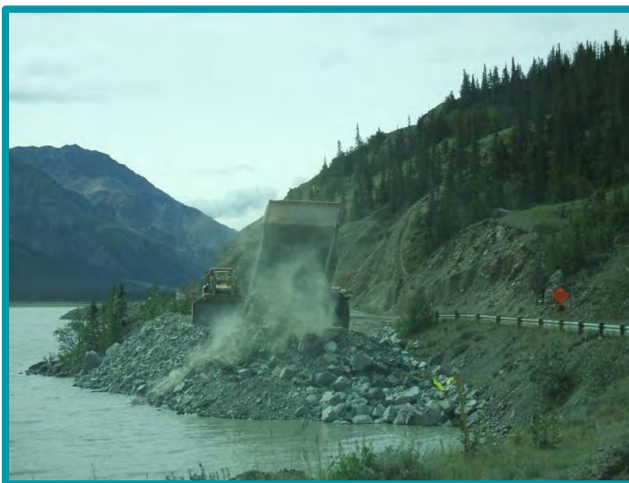
3.10-03 For this road-widening project, the lake edge had to be infilled. The procedure involved dumping rock on the ramp and then carefully push it into the lake with a dozer.
