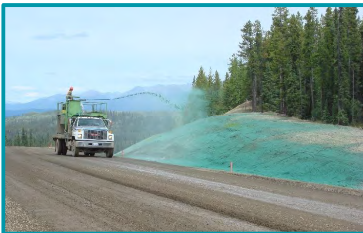
2.1.2-04 Hydroseeding in progress. The slurry sprayed onto the slope contains a wet slurry of a fibrous mulch, seed and fertilizer. A tackifier is often included so the mixture sticks together better.
