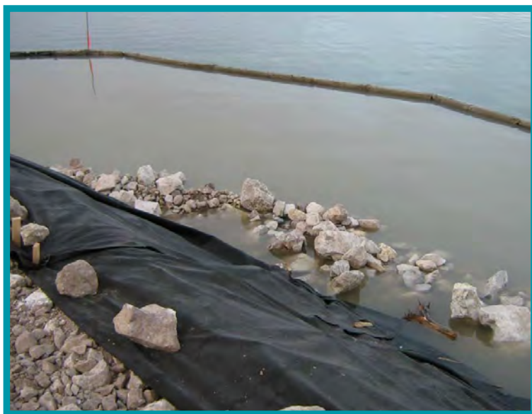
3.11-01 Little Atlin Lake boat ramp is being expanded. Infill area in the lake has been isolated with a silt curtain to contain sediment. Note the turbid water inside of the silt curtain compared to the remainder of the lake which is clear.
