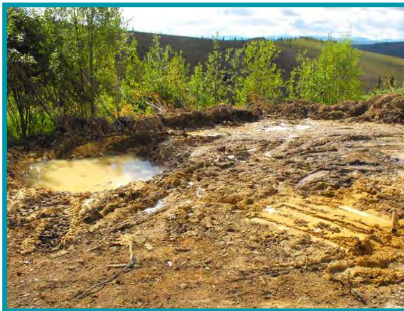
3.12-03 Decommission of this drilling pad is nearly complete. The sump remains and the site still needs to be reclaimed. Note the pile of organic material piled along the edge of the vegetation. This will be spread over the mineral soil and the site will be seeded.
