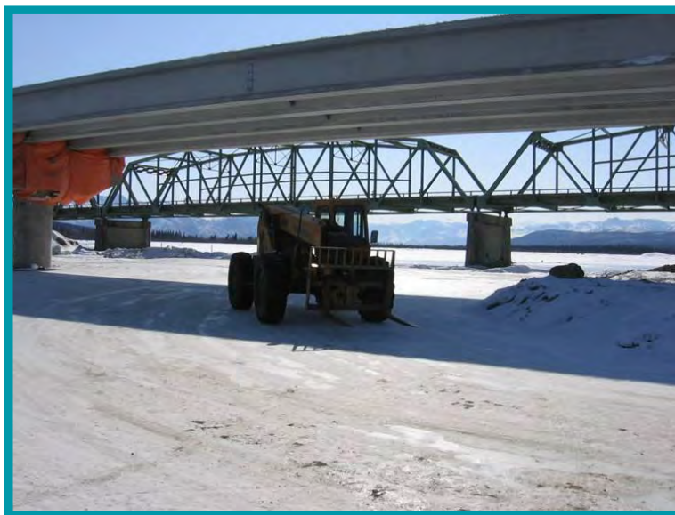
3.7-01 Working from the ice is often a preferred way to access the underside of bridges, and makes it much easier to protect water bodies. In this case, an ice bridge across the Donjek River was built to facilitate construction of a new bridge.
