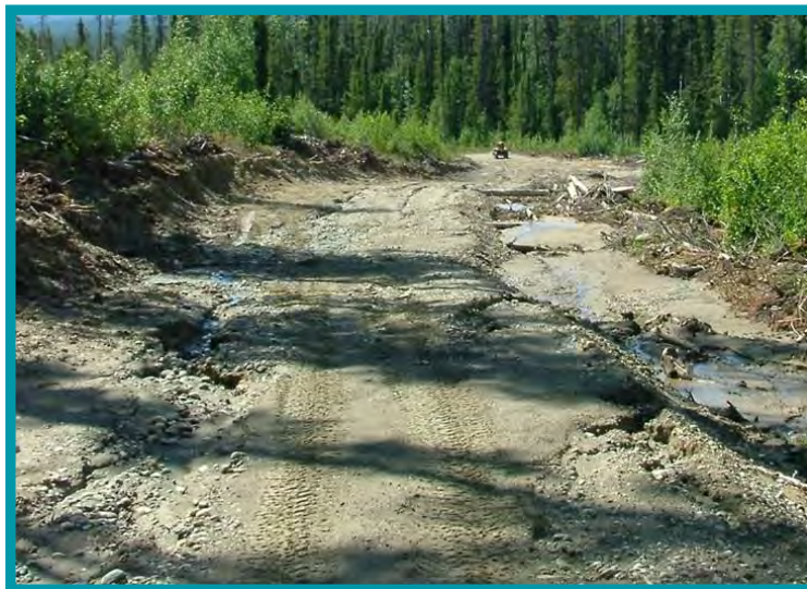
3.3-01 The lack of drainage control on this road has resulted in major washouts and has made the road barely useable.
