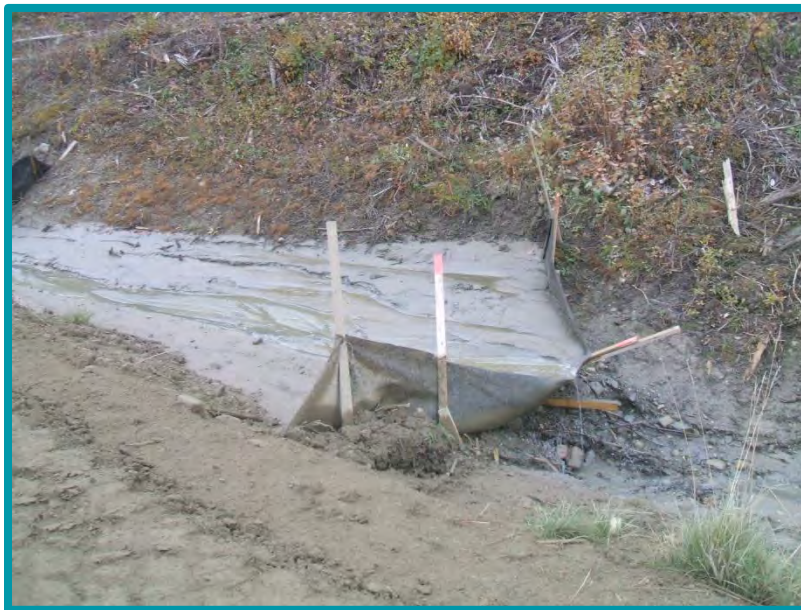
2.1.7-01 This silt fence illustrates that even an imperfectly implemented sediment control measure is better than nothing. The fence did its job, but could have been built better and it is beginning to fail. It is collapsing because of inadequate staking; metal rebar or larger wood stakes should have been used. Also, the fabric is unwoven geotextile cloth. Woven geotextile would have been a better choice, as it is stronger and will sag less. The fence will need to be cleaned out before it loses its usefulness.
