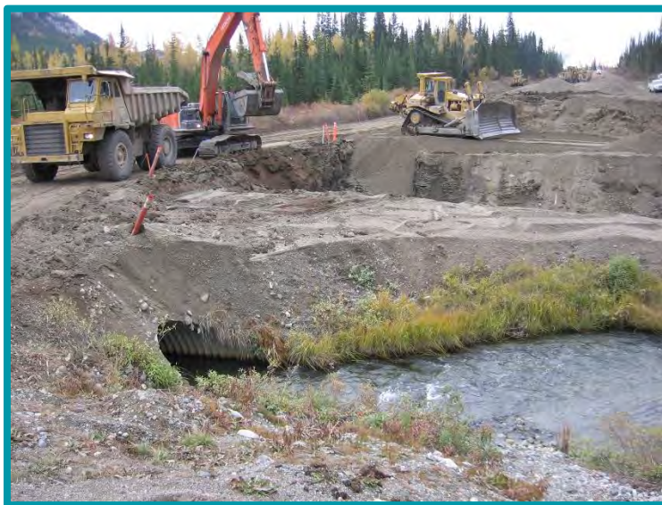
3.6-01 The site of a new culvert crossing is being prepared “in the dry”, while the stream is left undisturbed. The old culvert and channel will be reclaimed after the new one is activated.
