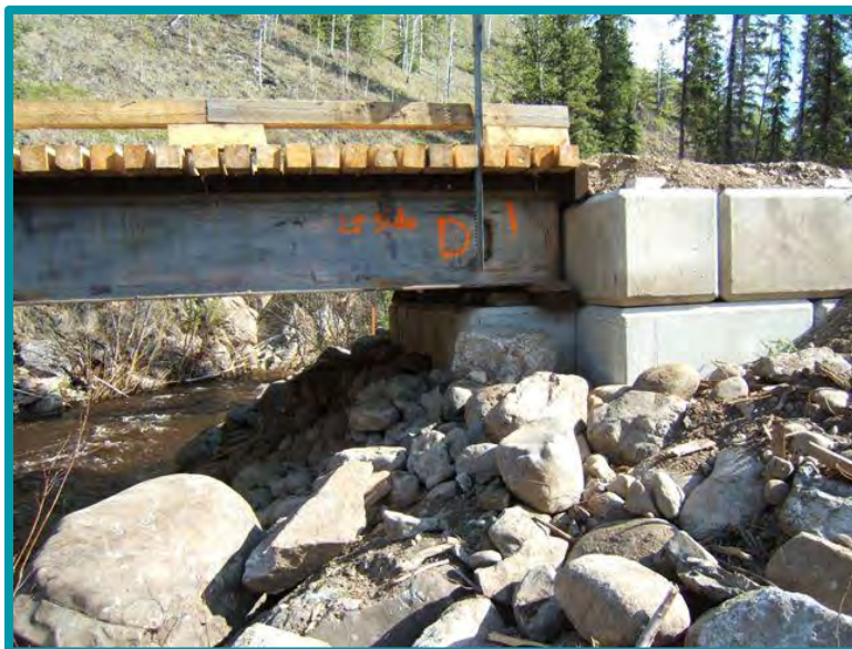
3.5-02 A properly-installed permanent clear-span bridge with riprap for bank protection.
