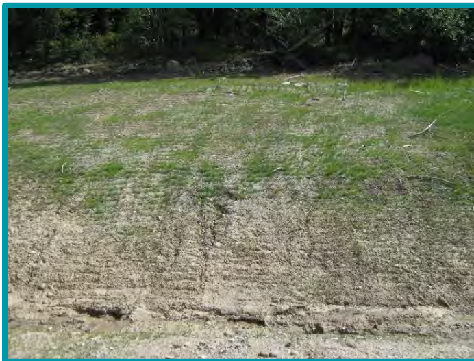
2.1.5-01 Slope tracking and seeding. This slope was nicely tracked with a Cat and seeded the year prior to taking this picture.
