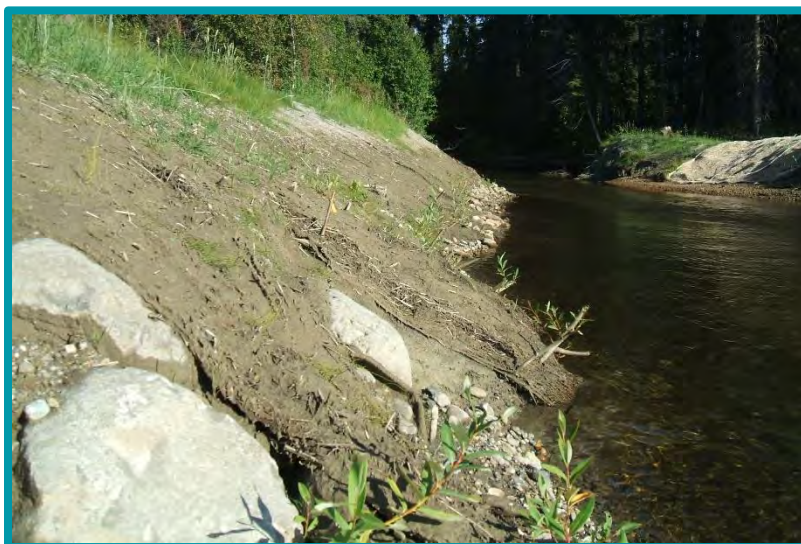
2.1.4-02 The same site as in photo 2.1.4-01 one year later. Grass is emerging and the willow cuttings are growing along the water. The slope may look exposed and prone to erosion, but the buried erosion control project is keeping the slope stable while vegetation becomes established.
