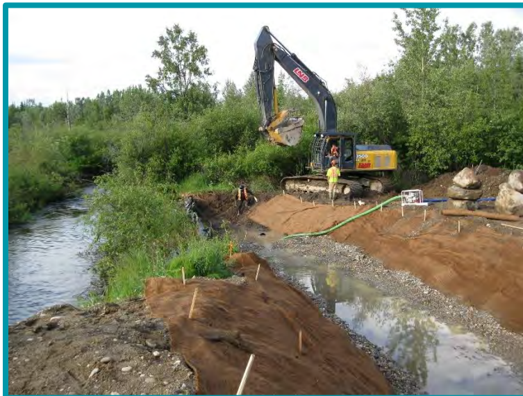
3.8-03 The project in the following six photos involved lengthening two existing culverts at Watson Creek. To complete the work, the creek had to be diverted so the culvert extensions could be completed in the dry. This photograph shows the diversion channel on the right and Watson Creek on the left. The banks are lined with jute fabric to protect them from erosion. The new channel is being washed and the sediment-loaded water is being pumped out into the vegetation.
