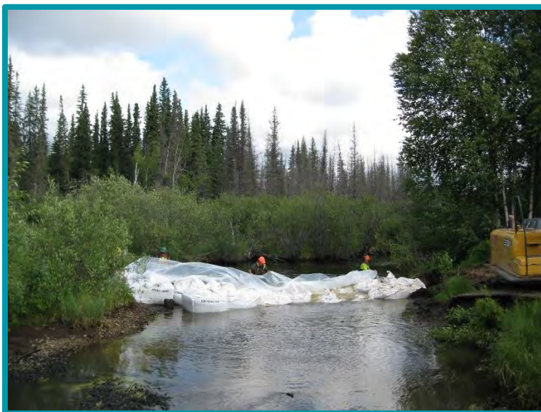
3.8-07 Same site - the sand bags are covered with plastic on the upstream side of the diversion. The plastic is anchored on the bottom with rocks to hold it in place and to seal the stream blockage.
