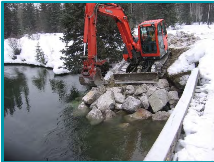
3.10-02 A temporary ramp consisting of large, clean rock infill was constructed so the excavator could access the stream and work underneath the bridge. After the work was completed, the rock was removed.
