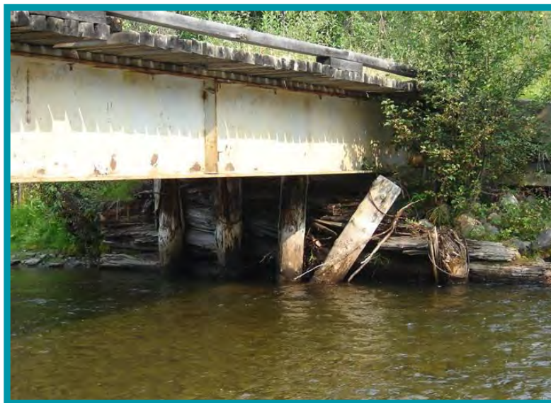
2.1.1-02 The abutment and approach (not shown) of this bridge failed because surface drainage water flowed to the bridge rather than being directed away from it. This could easily have been prevented with proper grading and bridge design.
