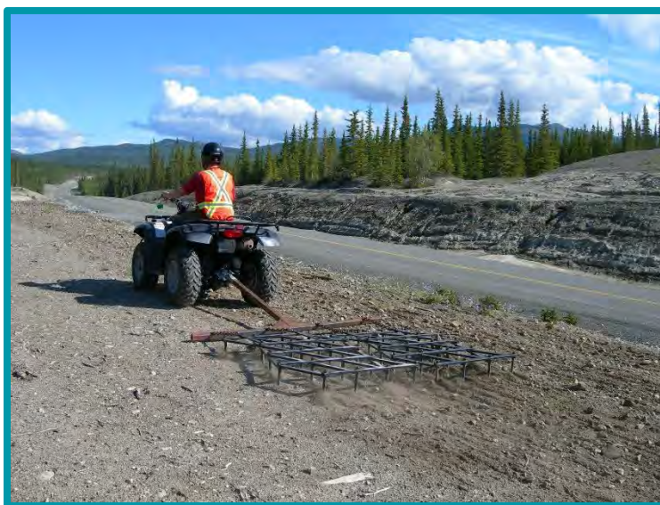
2.1.2-05 Soil preparation. The surface is loosened with a tine harrow prior to seeding. Many large seeding projects can be completed by a two-person crew using an ATV equipped with a harrow and broadcast seeding, in conjunction with hand seeding.
