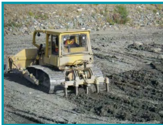
2.1.5-02 Extreme roughening of the surface with a ripper.
