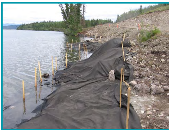
3.2-02 All that was available on short notice as a temporary erosion control measure on this road building project was unwoven geotextile cloth. While not the preferred material, this impromptu action on the part of the contractor was a resourceful solution, and was well-executed (note the ample staking). A week later, the permanent solution was installed that consisted of large rock (riprap) placed along the bank.
