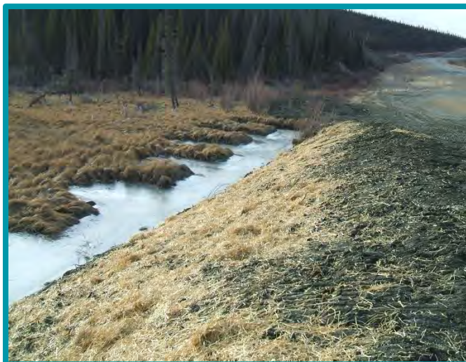
2.1.3-01 Straw mulch used on a stream bank to protect a seeded from erosion. This straw should have been worked into the ground surface better so it will not blow away or wash into the water body.
