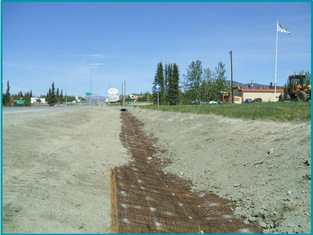
2.1.4-03 Coconut fibre matting reinforced with a UV resistant mesh was installed in a ditch that was prone to erosion and had a direct outlet into an adjacent river. The site was seeded prior to installation of the matting. There are two installation errors to note: the edges of the matting should have been folded into the side slopes by means of creating an anchor trench, rather than lying flat on the ground. Also, no dirt should have been put on top of the matting.
