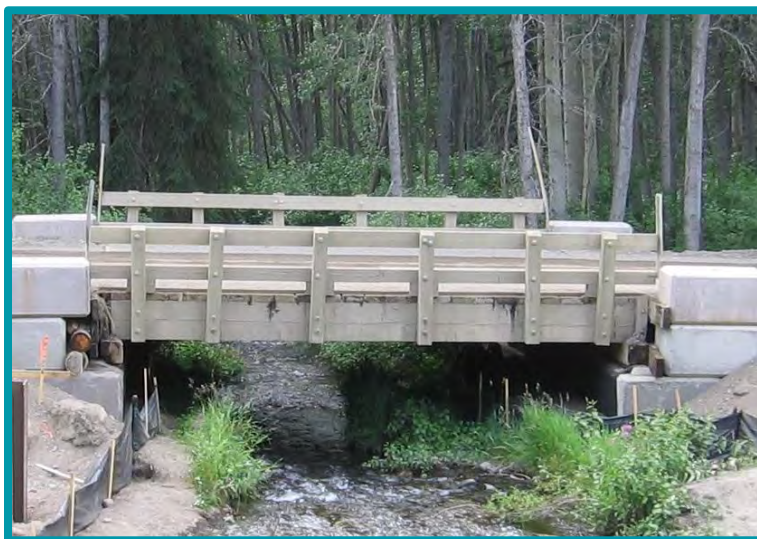
3.5-01 A properly-installed temporary clear-span bridge with perimeter silt fences.
