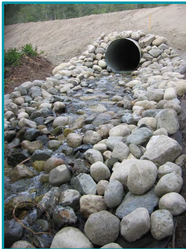
2.1.1-03 Rock flume. A rock flume is an erosion control measure commonly used for culvert outlets located on steep grades.
