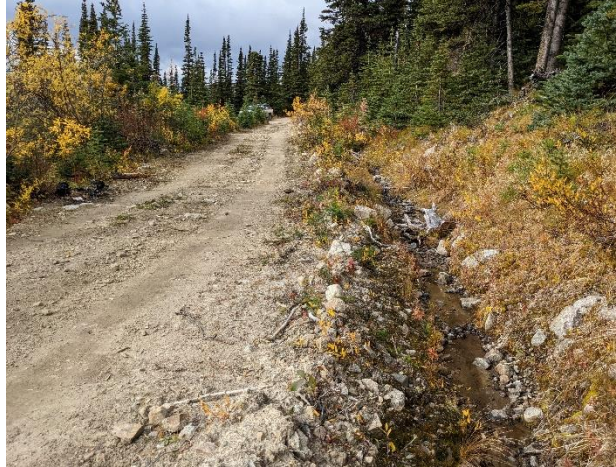
Photo 10. CMC-SS flow travelling along ditch on south side of site. WRB crew dug a small hole to allow for sampling then returned several hours later to collect sample after stirred sediment had flushed.
