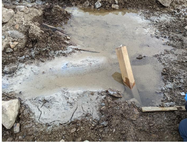
Photo 8. CMC-BH2. Piece of 4"x4" lumber inserted into ground, material which appears to be bentonite present on ground surrounding hole. Nearly undetectable flow <1 L/s.
