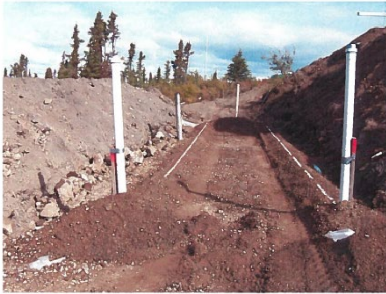
Photo 1. Taken from Waterline as-built documents (EBA, 2008), and described as “placement of 40mm crushed gravel mounded on either side of the PVC pipe prior to placement of geotextile (August 18, 2008)”.
