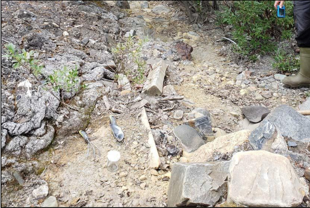
Photo 3. Sample site ONEK-S2 in the discharge channel below the Wernecke Road culvert.
