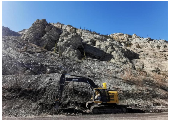
Rock trenching crew, preparing for conduit installation.
