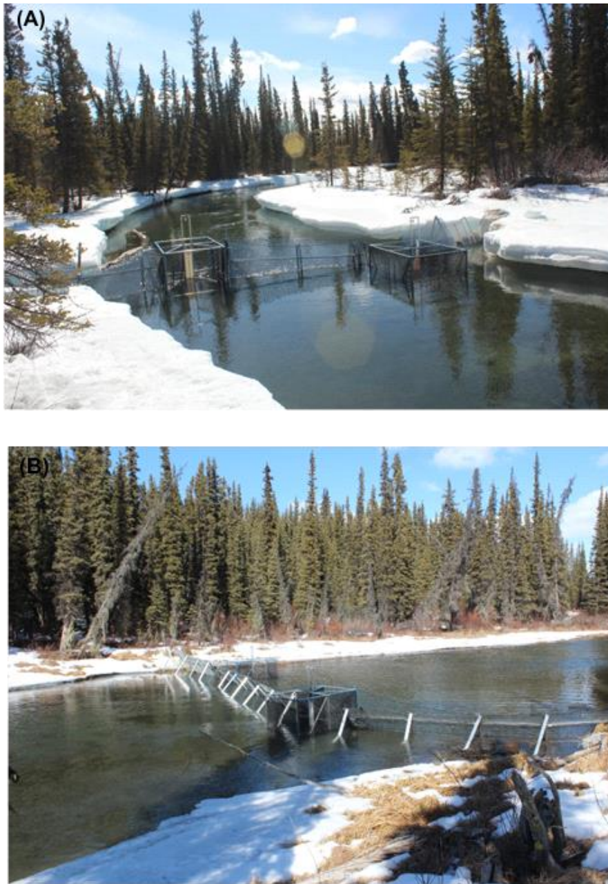
Figure 2. The general weir construction used for assessing the Lubbock River spawning population. Images show the downstream weir (A) and the upstream (Little Atlin Lake outlet) weir (B). Both weirs were in place for the duration of the spawning period (April 27 and July 2).
