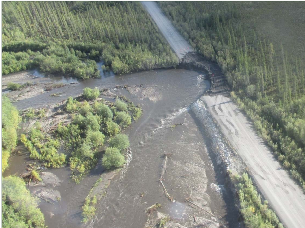
Photo 1-3. Erosion of the Dempster Highway embankment following a high-intensity, mid-summer rain event in August 2016 (photo credit: YG Highways and Public Works – Transportation and Engineering Branch [HPW-TEB])
