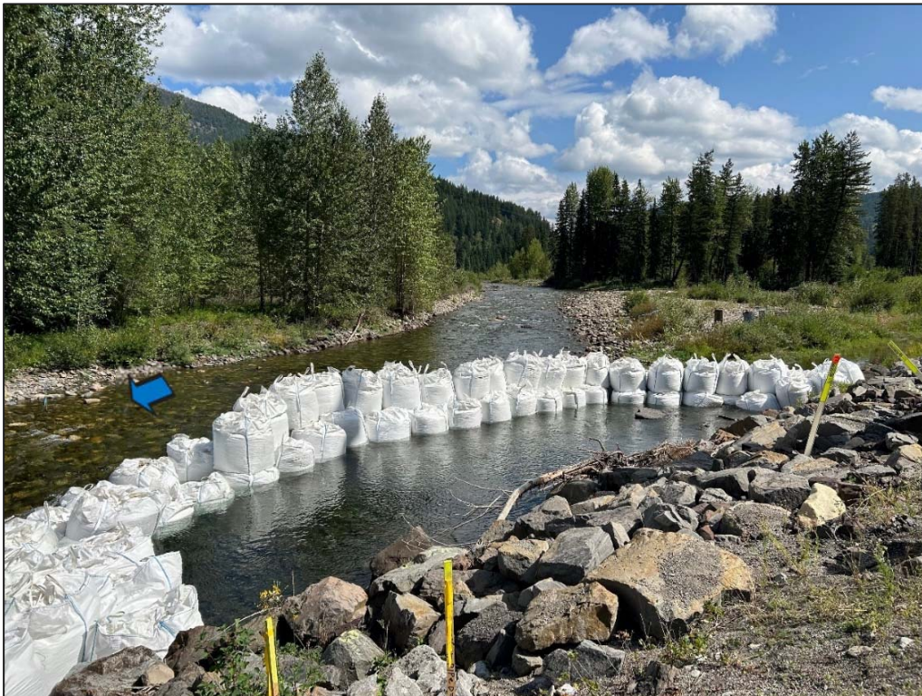
Photo 4-12. Example of site isolation along river using meter bags (photo credit: SLR). Note that the work area remains ‘wet’, but any sediments that become suspended within the work area cannot escape into the adjacent, flowing channel.
