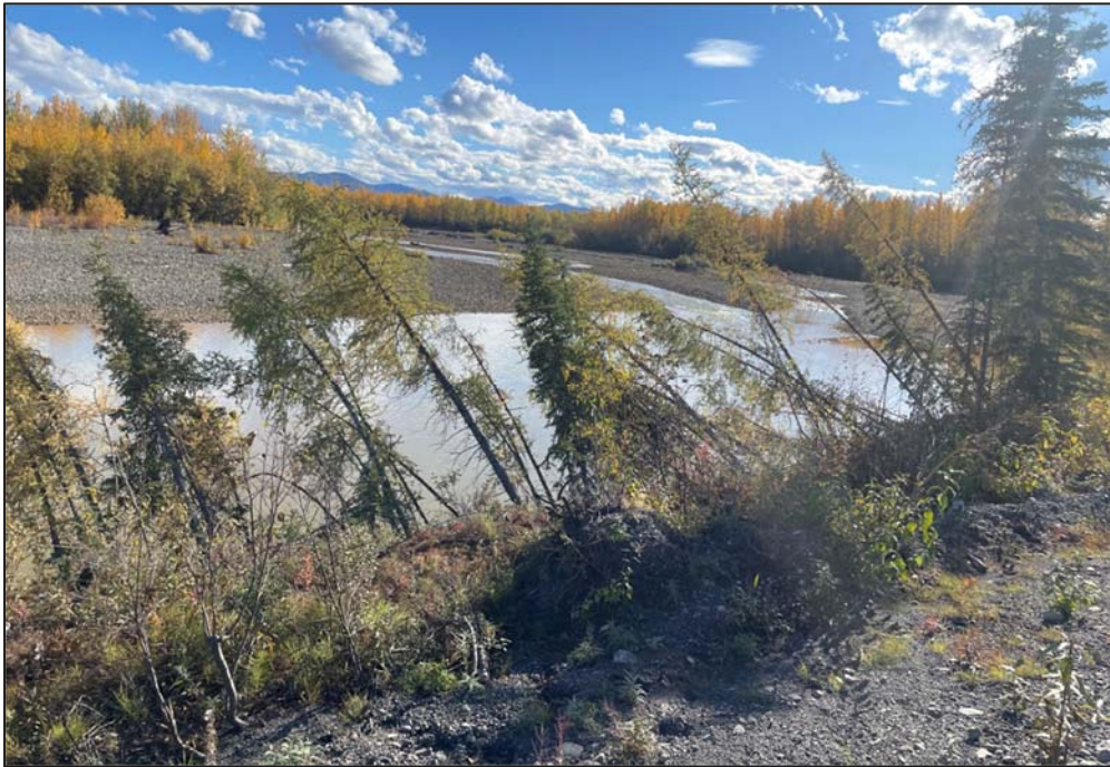
Photo 5-1. An eroding bank of a watercourse is within a few metres of the road embankment (photo credit: SLR). Although not truly an emergency, this site may be classified as urgent as a large flow event may lead to a road washout.
