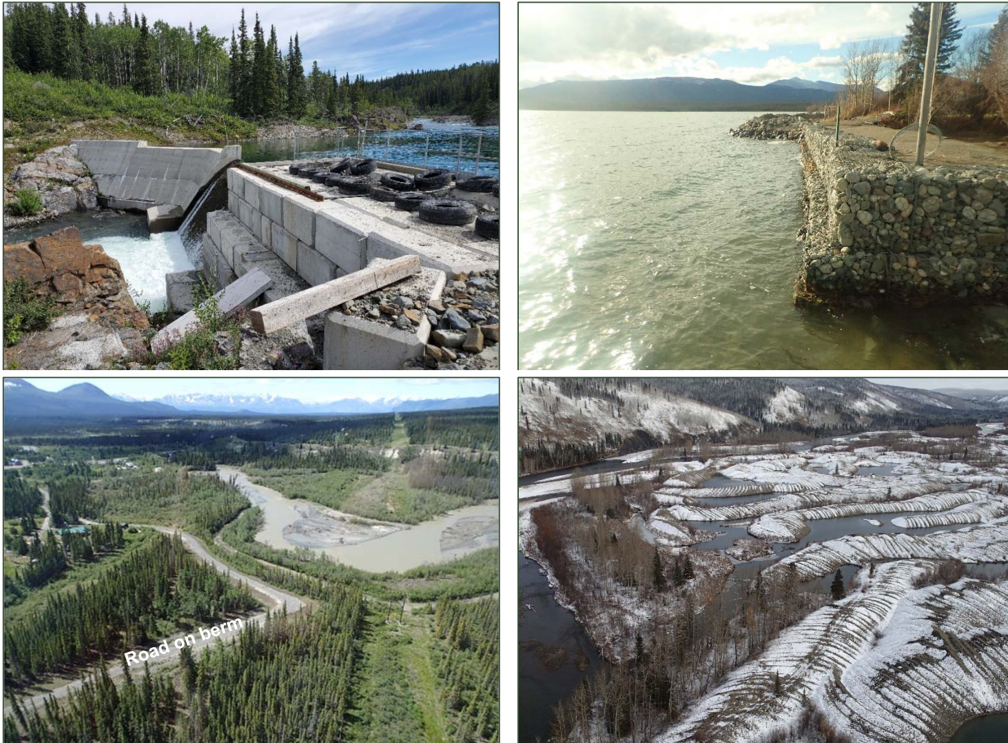
Photo 2-10. Examples of anthropogenic influences. Top left: a hydro-electric flow control structure at Surprise Lake near Atlin, British Columbia (photo credit: SLR). Top right: gabion basket erosion mitigation structures on Marsh Lake (photo credit: Benoit Turcotte). Bottom left: anthropogenic berm protecting the village of Canyon (photo credit: SLR). Bottom right: historical placer mining tailings alongside Klondike River near Dawson (photo credit: SLR).
