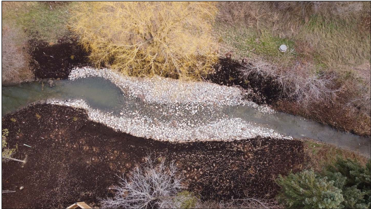
Photo 4-15. A UAV inspection of recently completed erosion mitigation works (white area of cobble riffle between regraded banks), including site restoration and riparian plantings (dark brown areas of freshly placed topsoil, mulch, and plantings) (photo credit: Toronto and Region Conservation Authority).
