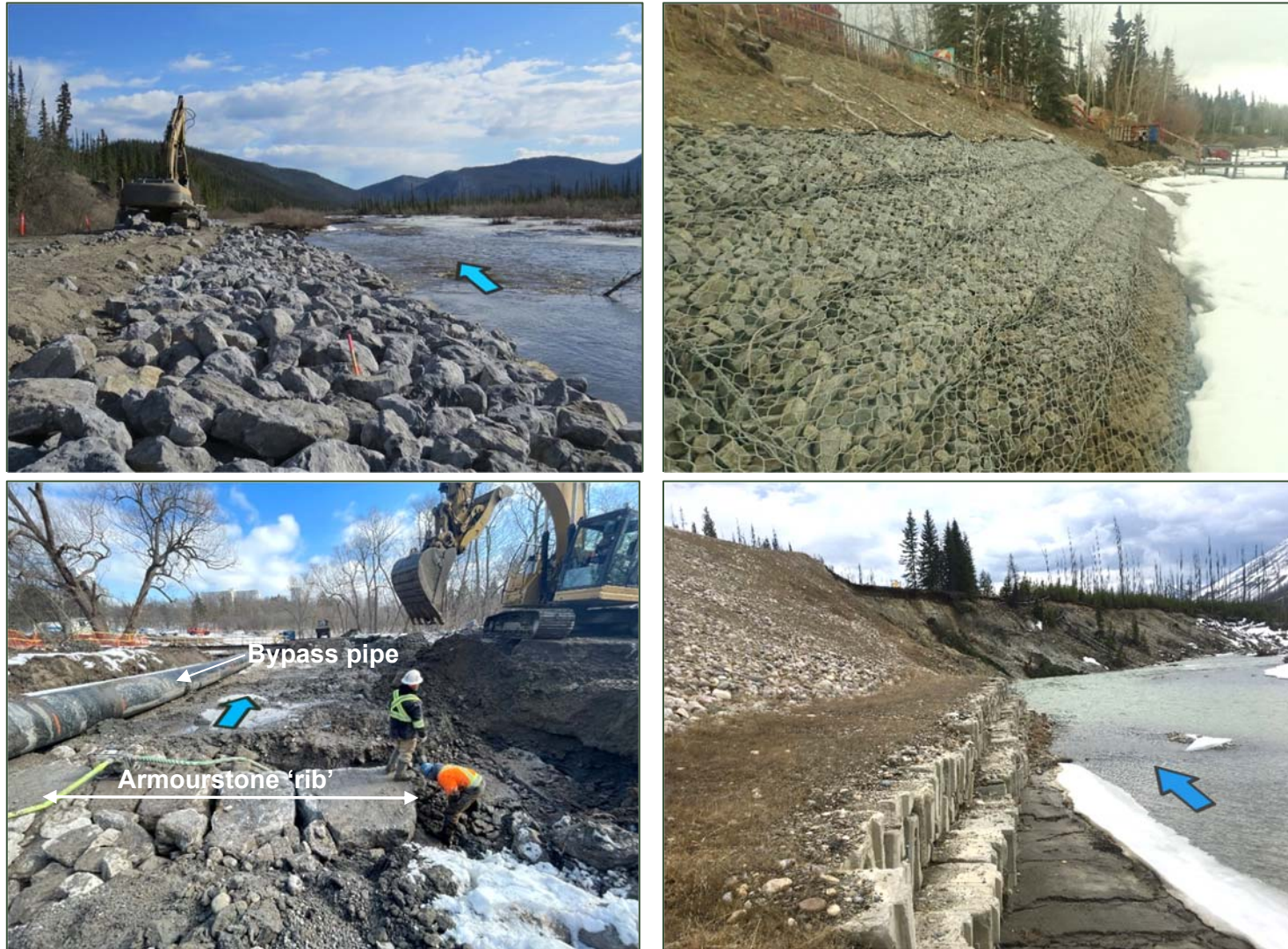
Photo 4-6. Examples of direct approaches to erosion mitigation. Top left: riprap embankment along the Dempster Highway (photo credit: YG HPW-TEB). Top right: gabion baskets along a lakeshore of Marsh Lake (photo credit: Benoit Turcotte). Bottom left: armourstone 'ribs' to protect buried sewers in Toronto, Ontario (photo credit: SLR). Bottom right: armourstone and riprap embankment in Kootenay National Park (photo credit: SLR).
