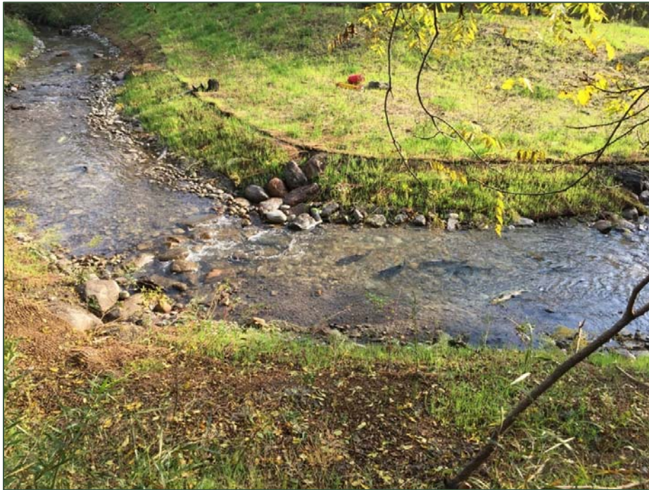
Photo 4-4. A small rock weir constructed to help dissipate energy and provide ecological benefit (photo credit: SLR). The weir was constructed as part of a larger channel realignment project in the Greater Toronto Area to reduce toe erosion along a failing slope near residential properties.
