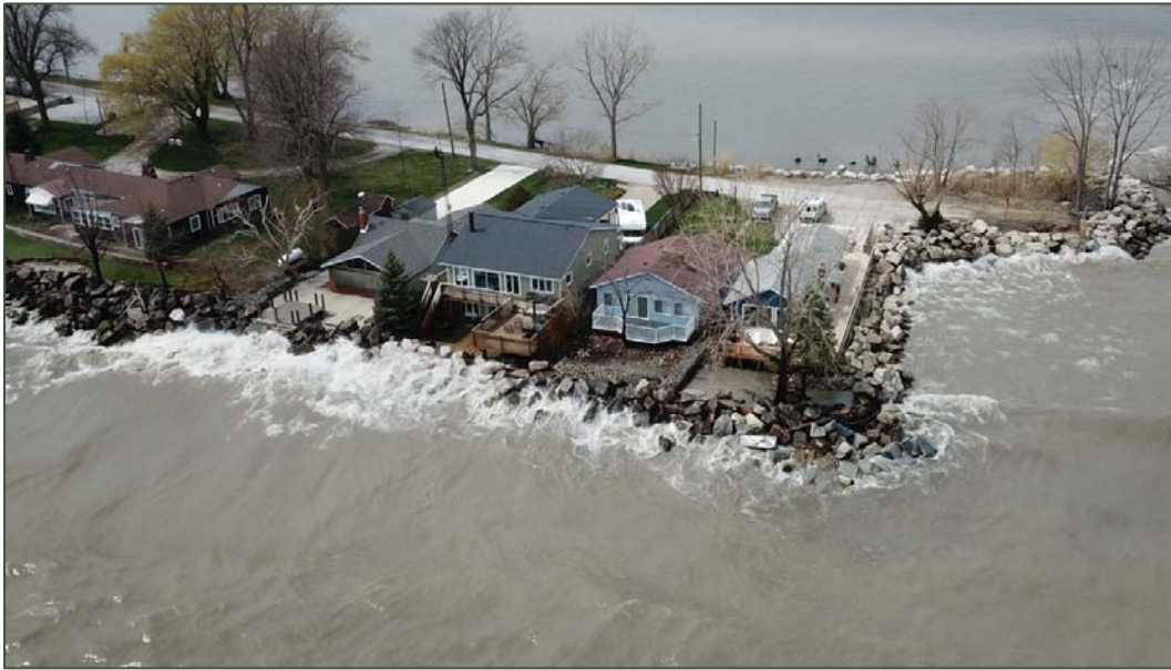
Photo 1-4. Waves breaking along a lakeshore armoured with large riprap to help protect private properties on Lake Erie (photo credit: SJL Engineering Inc. [SJL])
