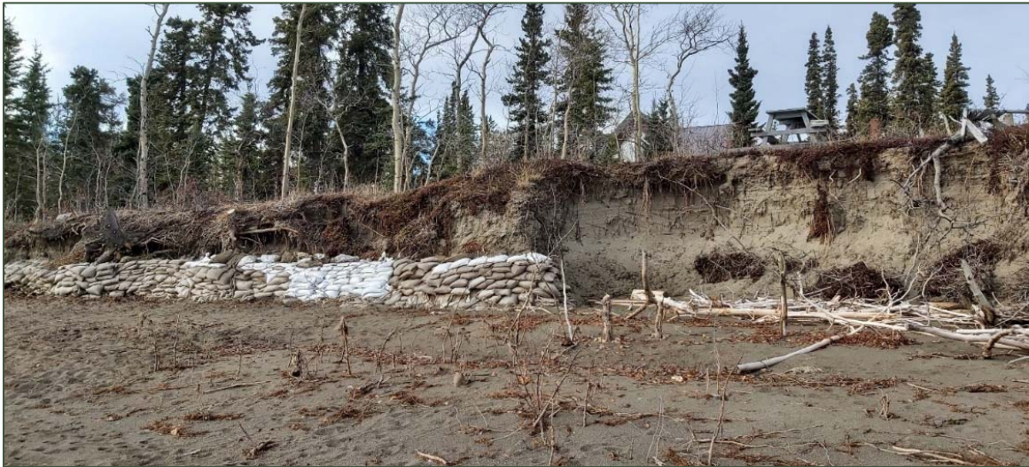
Photo 1-2. Erosion and temporary erosion mitigation materials along the shoreline of Marsh Lake (photo credit: Benoit Turcotte)
