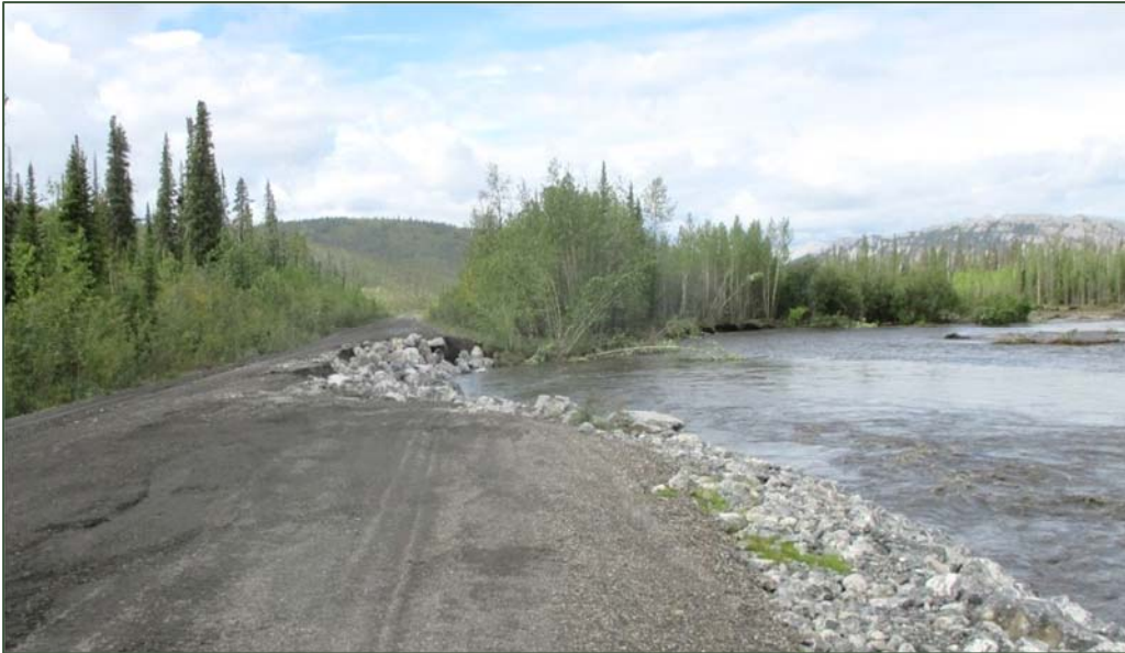
Photo 4-2. Temporary erosion mitigation following a road washout along the Dempster Highway during the August 2016 flood (photo credit: YG HPW-TEB). The temporary measure does not negate the need to reconstruct the highway, but it minimizes the service disruption by allowing alternating traffic to pass until the highway is reconstructed.
