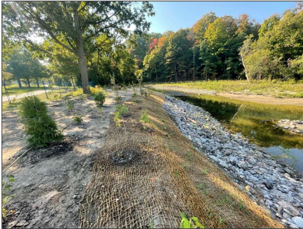
Photo 4-13. An example of site restoration including soil stabilization coir matting and riparian plantings (photo credit: SLR).
