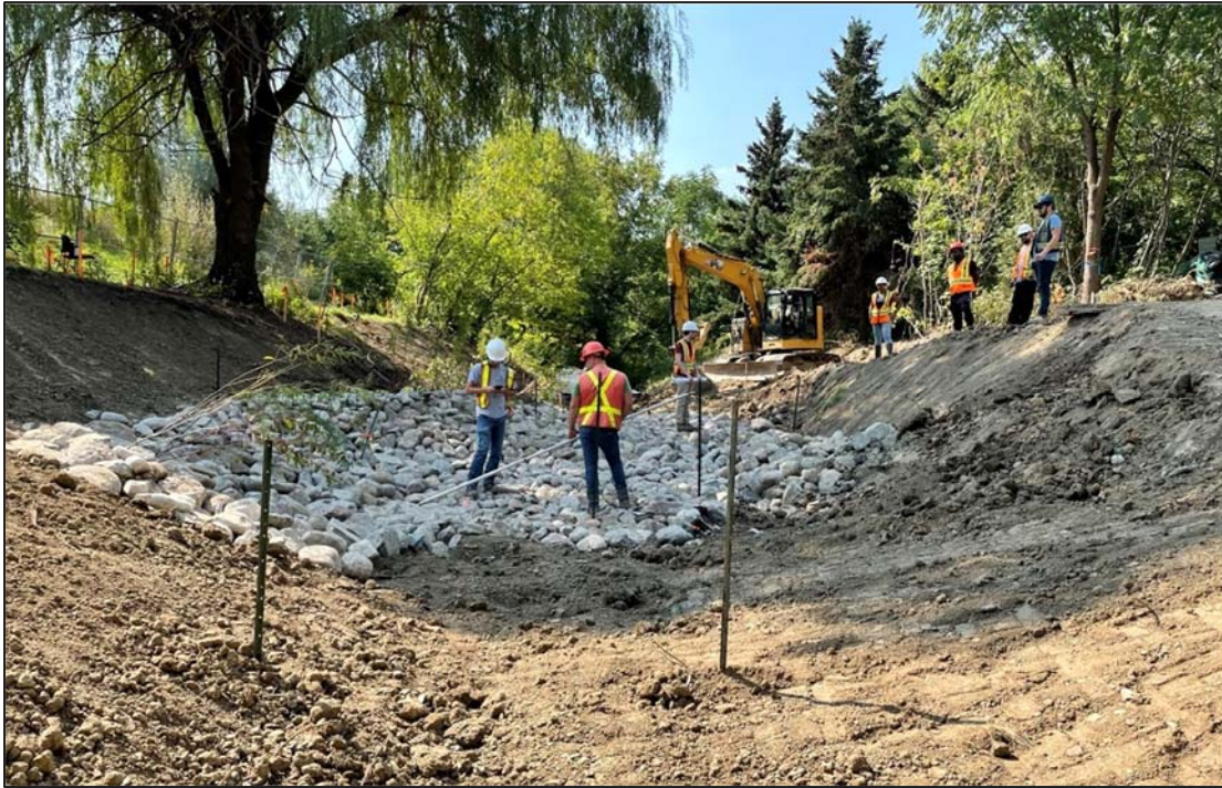
Photo 4-14. Inspection of completed erosion mitigation works by members of the design team, along an isolated (dry) section of watercourse, prior to advancing to the next phase of construction (photo credit: SLR).
