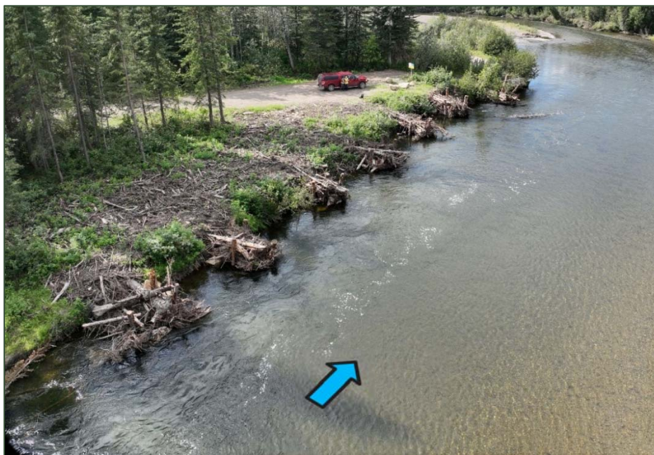
Photo 4-5. Constructed wood 'spurs' along Mayo River that deflect erosive energy away from the riverbank (photo credit: Ecological Logistics and Research Ltd.).
