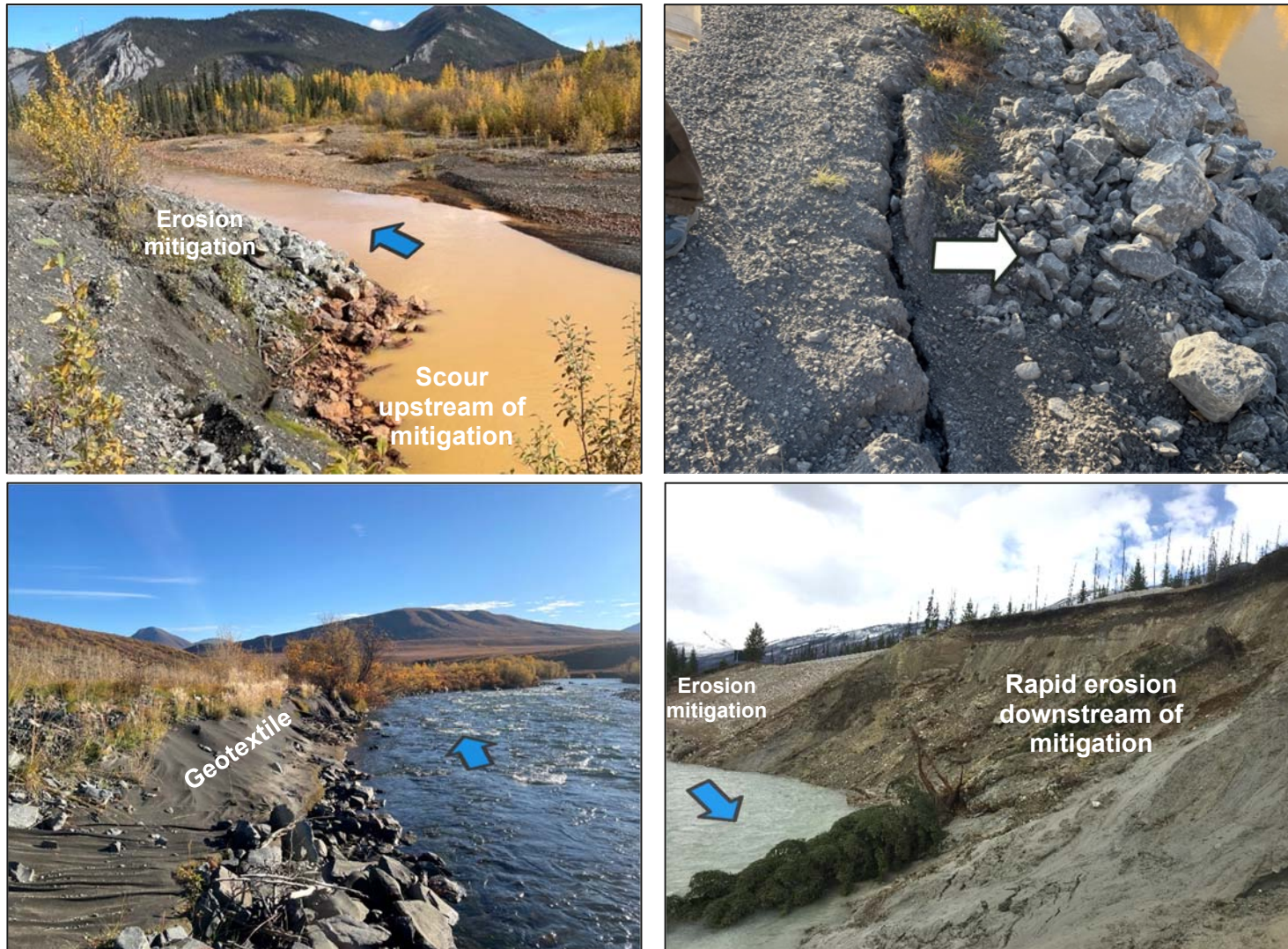
Photo 4-17. Examples of common reasons for erosion mitigation failure. Upper left: riprap embankment was not extended far enough upstream. Upper right: riprap was not adequately embedded, contributing to slope failure. Bottom left: geotextile created a slip plane for riprap. Bottom right: erosion protection was not extended far enough downstream. All photos courtesy of SLR.
