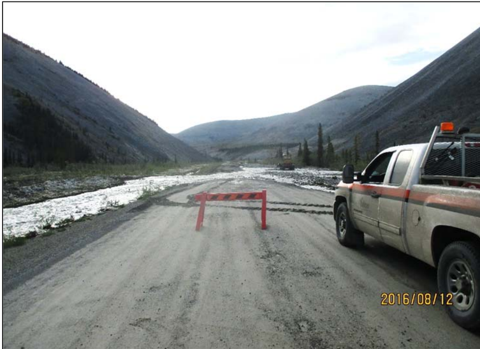
Photo 4-9. Following a high-intensity precipitation event in August 2016, a watercourse severed the Dempster Highway and necessitated emergency works to allow for safe passage of vehicles transporting critical supplies between communities (photo credit: YG HPW-TEB).
