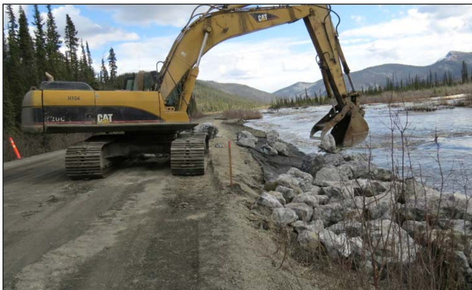
Photo 4-11. Careful placement of riprap on an embankment using specialized equipment leads to better long-term results (photo credit: YG HPW-TEB). In this photo the riprap is being placed atop geotextile, which can form a slip-surface and contribute to revetment failure (see Section 4.6).
