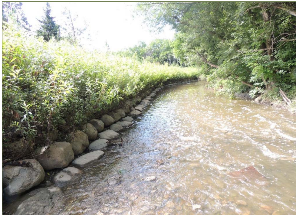
Photo 4-7. Extensive incorporation of native willows into riverbank erosion mitigation (photo credit: Toronto and Region Conservation Authority).
