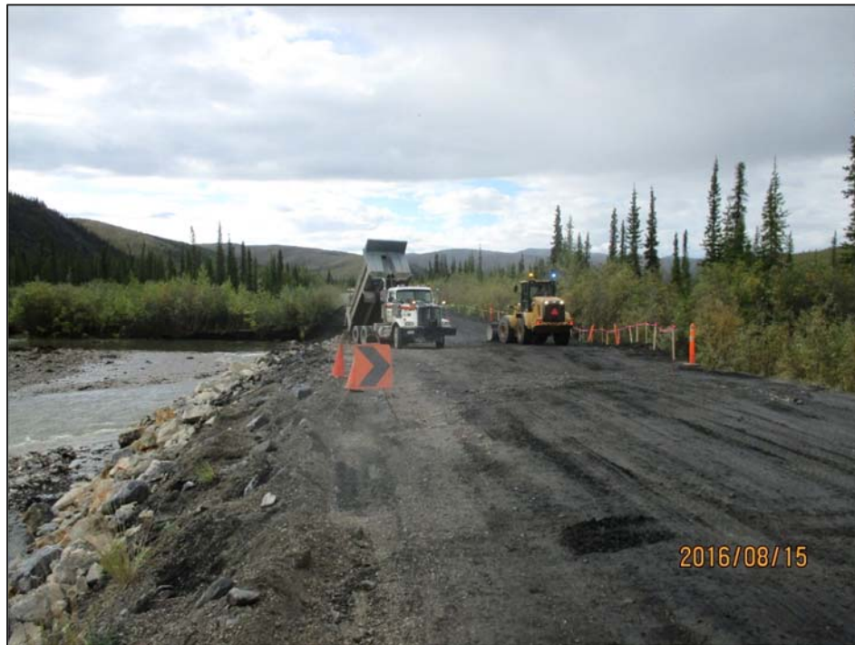
Photo 4-10. Emergency riprap installation utilizing end-dumping methods (photo credit: YG HPW-TEB). While expedient for rapid response, the lack of keyed placement and material segregation typically results in poor structural interlocking and limited long-term resilience.
