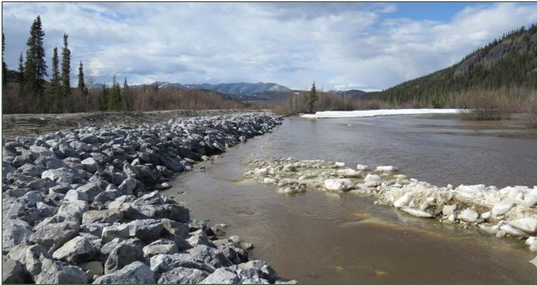
Photo 4-3. River ice interacting with recently constructed erosion mitigation along the Dempster Highway (photo credit: YG HPW-TEB).
