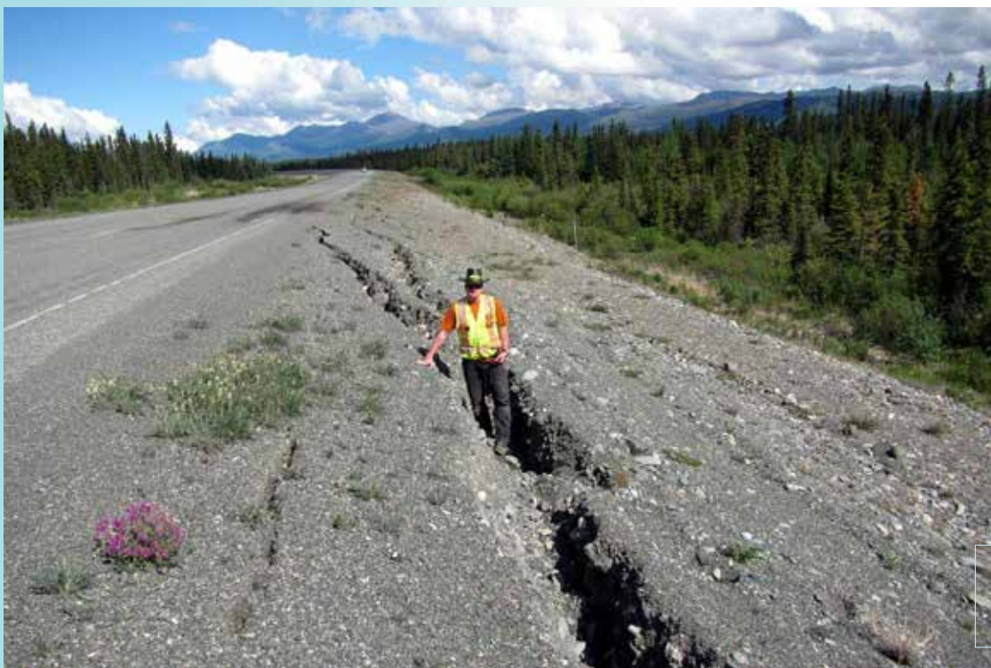
Cracks along the North Alaska Highway, 2013.
