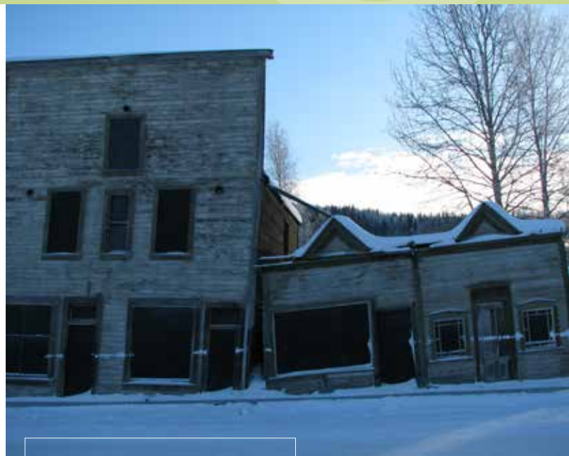
Buildings impacted by permafrost thaw in Dawson City.
