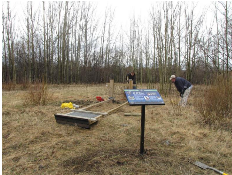
Figure 7. Bat house installation at Tagish Narrows Campground, Yukon.
