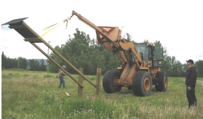
Figure 6. A loader is used to raise a bat house near Watson Lake, Yukon, in 2008.
