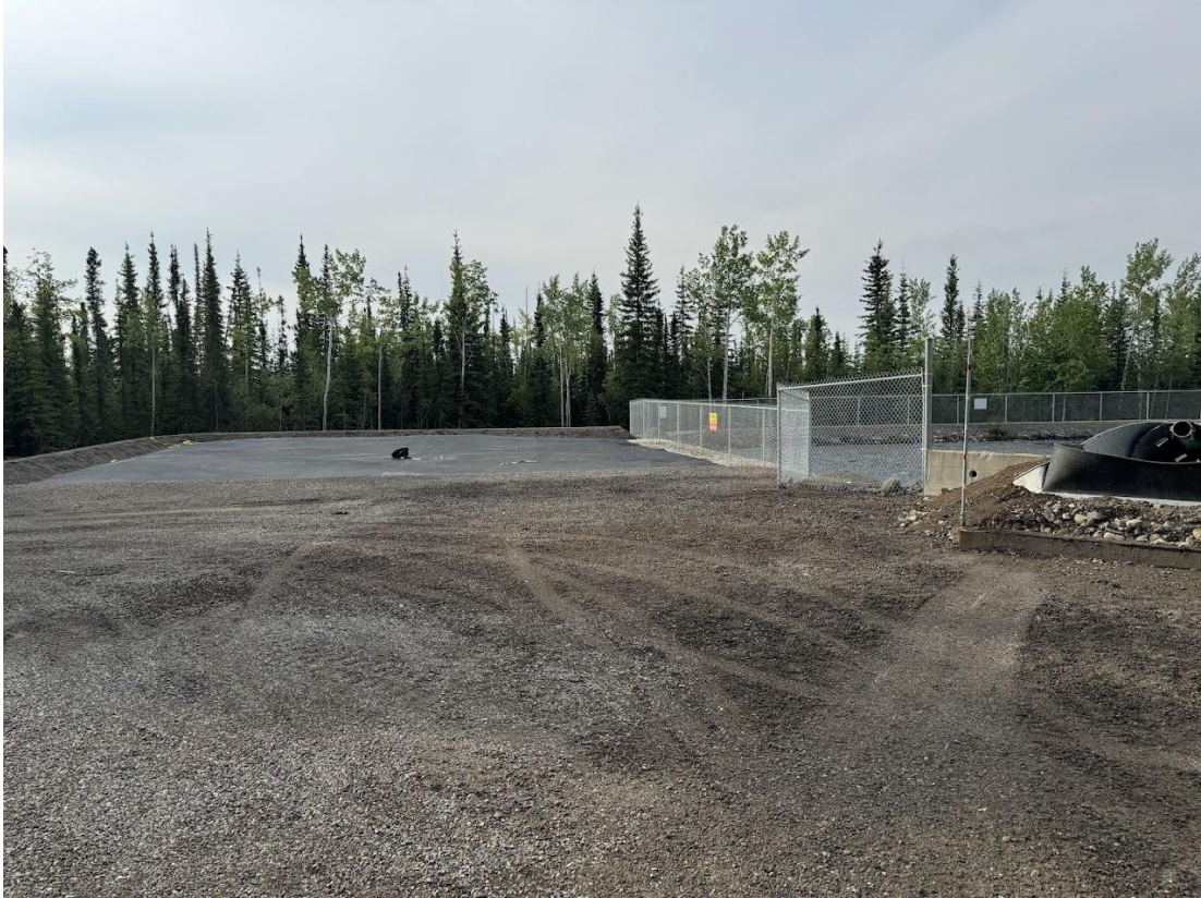
- Photo 4: Completed drying bed adjacent to the pit (WRB, June 24, 2023)
