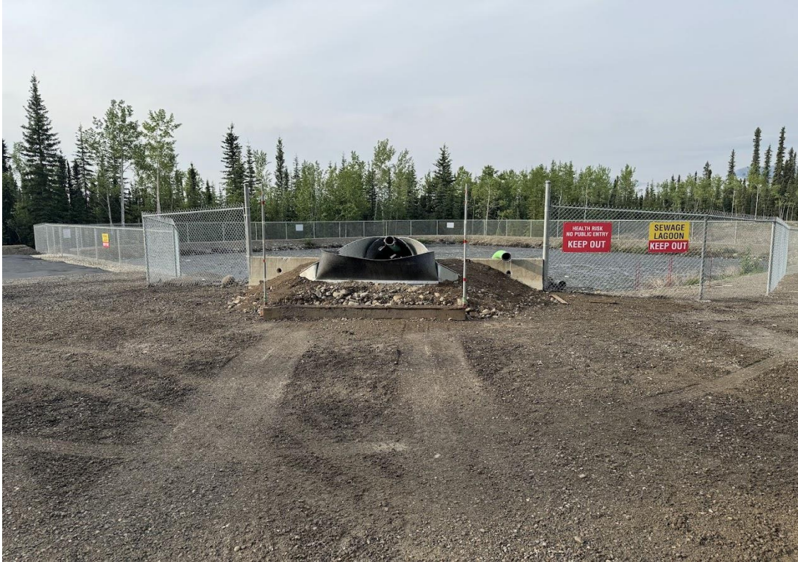
Photo 5: New fence and culvert installed at the pit (WRB, June 24, 2023)
