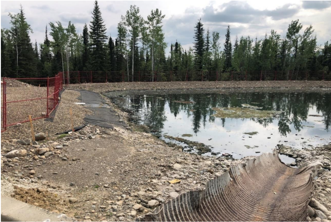
Photo 3: Partial view of the drying bed and the protruding PVC pipe on the left of the photo (WRB, June 7, 2023)
