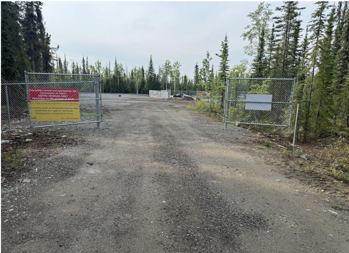
Photo 6: New site access gate installed (WRB, June 24, 2023)
